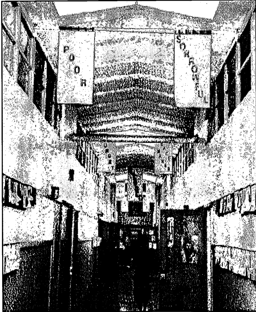
Figure 2. Central unconditioned hallway.
